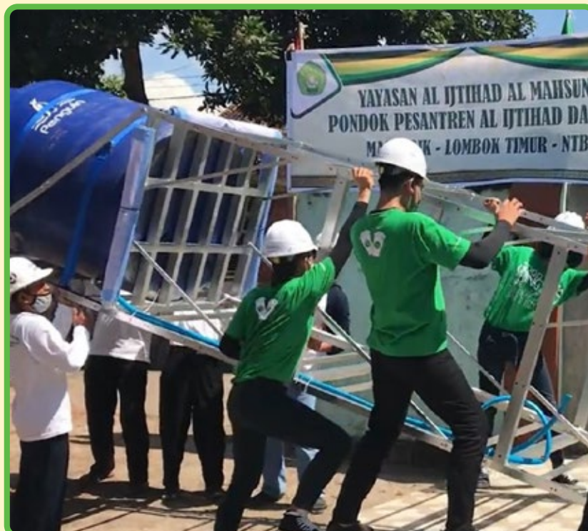
Installation of the 14 th water tower at Danger Village, East Lombok Pemasangan tower air ke-14 di Desa Danger, Lombok Timur
